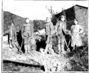
Detail, Schwab, Carr and others building shack
